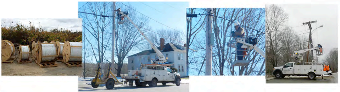
Construction of Petersham's broadband network continues
